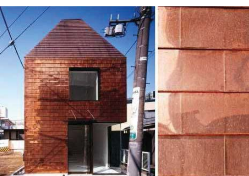
Metail shingles to roofs and walls
