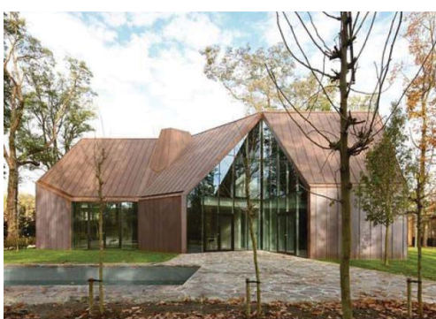
Standing seam pigmented zinc for roof and walls
